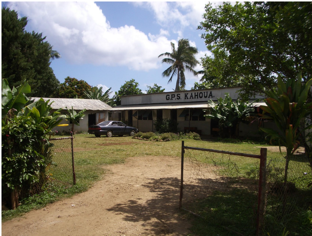
Plate 1: General view of site showing small size and both classroom buildings
