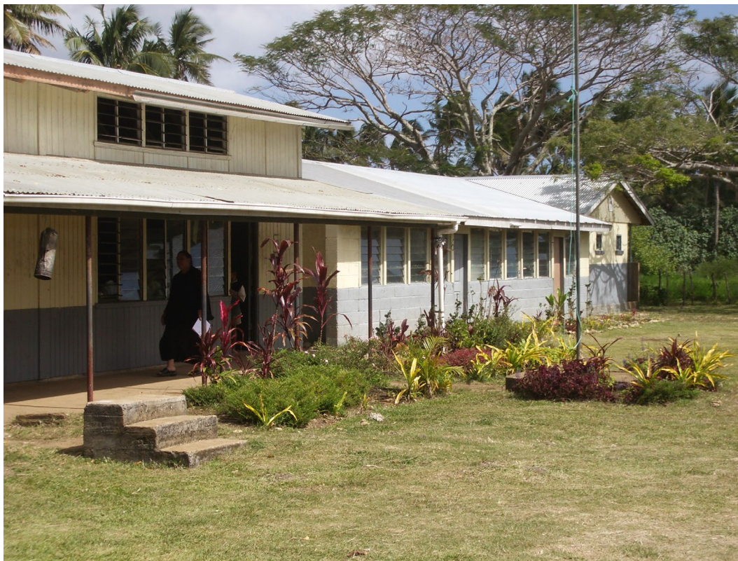
Plate 3: General view showing Classroom Buildings 1 and 2 and toilets at rear. Note low roof height of Classroom 2.
