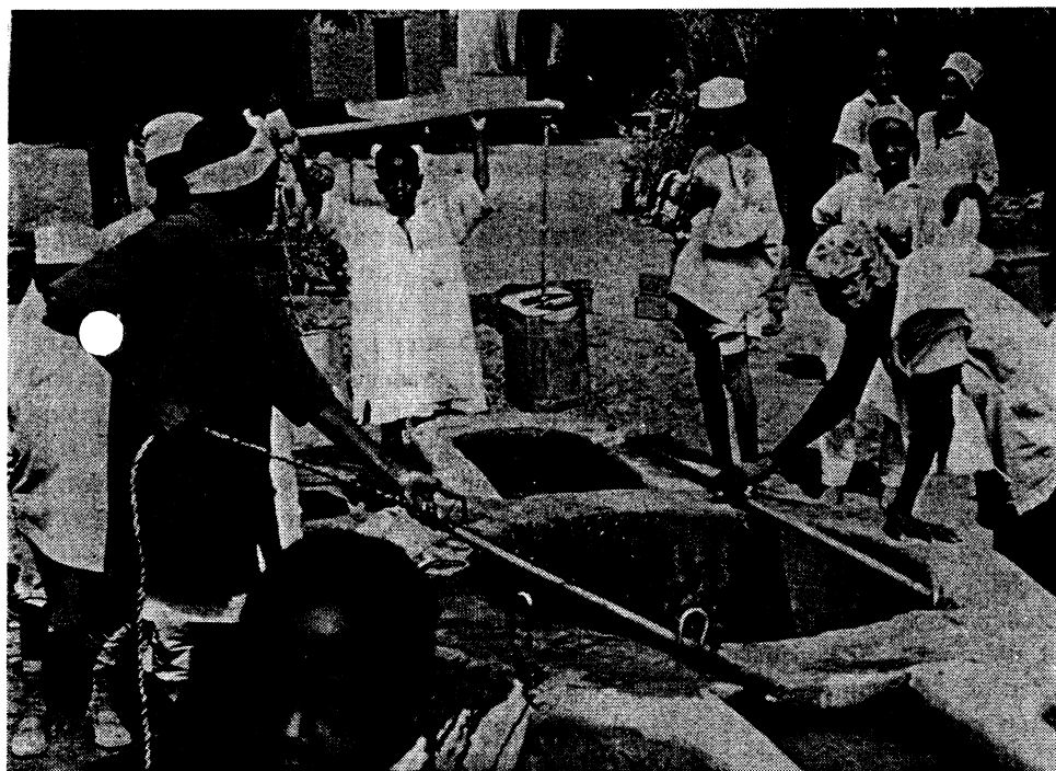
Figure 6 An open well with headwall. Note the metal bars used as rollers, which reduce the need to stand on the headwall to lift buckets. The basins at each side are for watering animals.
