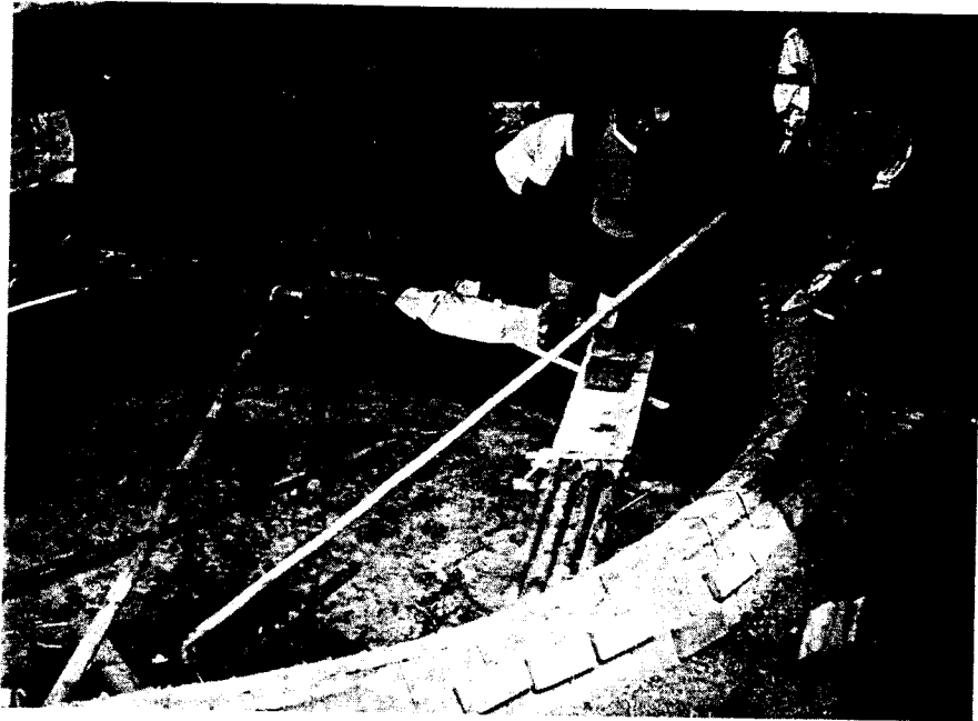
Fig. 58. Fixed dome biogas plant for cattle dung, under construction by CYSD and BORDA at a farm in Orissa / India [photo: Sasse]
