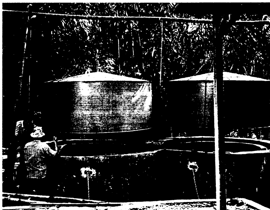
Fig. 57. Floating drum plant. The drums are lifted for re-painting which allows a view on the double ring wall of the water jacket. Constructed by LPTP and BORDA for a slaughter house in Java / Indonesia. [photo: Sasse]
