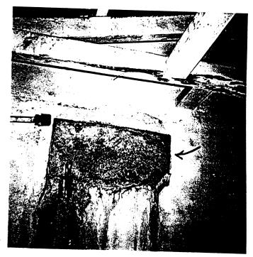
3.10k Sometimes basins or sinks are supplied with tap holes, but if only one tap is fitted the other hole or holes are left open. These can allow water to drip onto the floor below and are difficult to clean:
