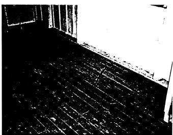
3.7h Timber WC and shower floors commonly get wet and rot from spilled showers and overflowing toilets. Such floors are not dangerous unless they are left for a long time during which they will become weak, collapse and encourage insects and mosquitoes so must be totally replaced. The floor structure under a wet area floor may also be damaged so must be inspected and repaired if necessary. there several steps:
