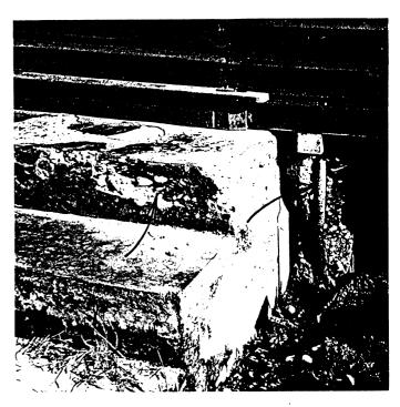
3.3g Concrete walkways that fall towards walls will trap rain, allow slippery mould to grow underfoot and encourage mosquitoes to breed. Incorrect falls must be fixed. the same applies to concrete floors that fall away from floor drains:
