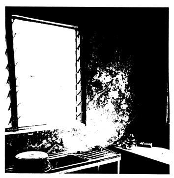
3.12e Damp parts of a building always encourage the growth of mould especially in the corners, the bottoms of walls and on doors especially in showers and toilet areas. This is unhygienic, encourages mosquitoes and must be cleaned regularly:
