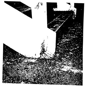
Door handles will often damage the wall lining behind them, or be damaged themselves because there is nothing to stop the door hitting the wall:
