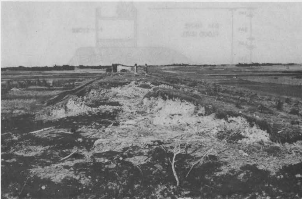
Plate 3. Part of the embankment along the coast and estuaries of Bangladesh. The cyclone of 1970 resulted in a storm surge which raised water over the embankment, washing away the part shown in the foreground.
