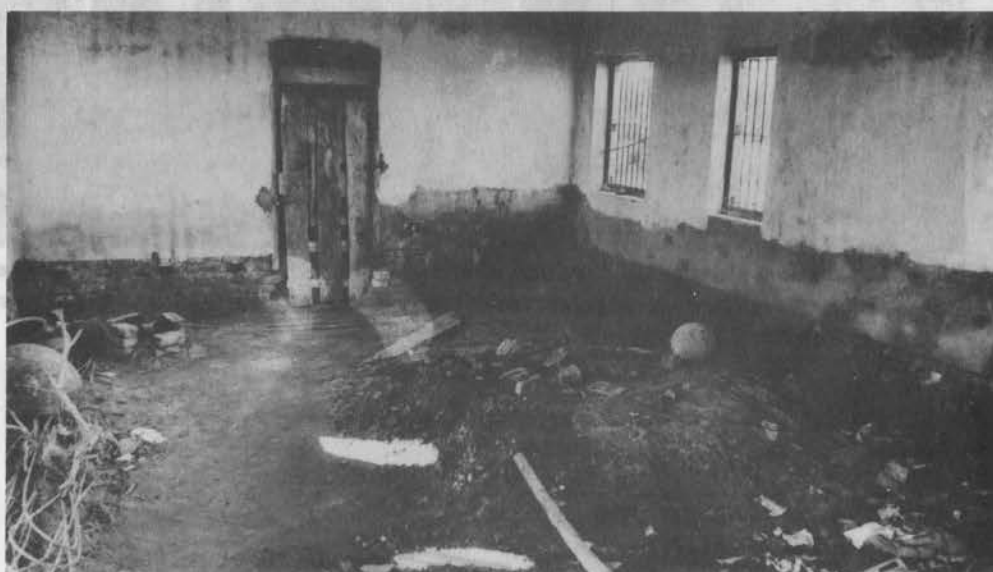
Plate 10. Mud and debris entrapped in a classroom after the subsidence of the storm surge waters of the Bangladesh 1970 cyclone
