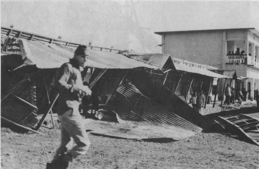
Plate 14. Inappropriate and inadequate use of corrugated galvanized iron causes frequent failures.
