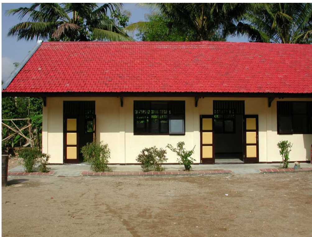
Plate 15: MIN Bungur showing new building
