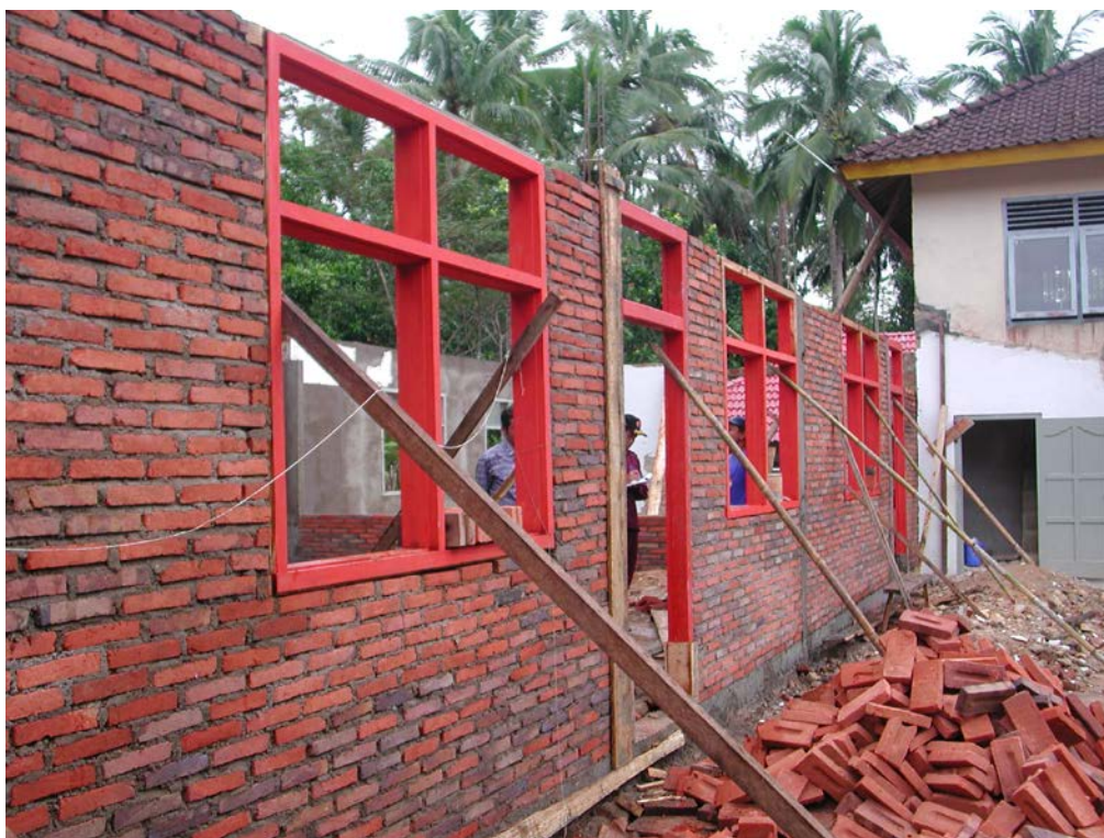
Plate 11: MTs Muhammadiyah 3 Ketro showing work in progress on classrooms
