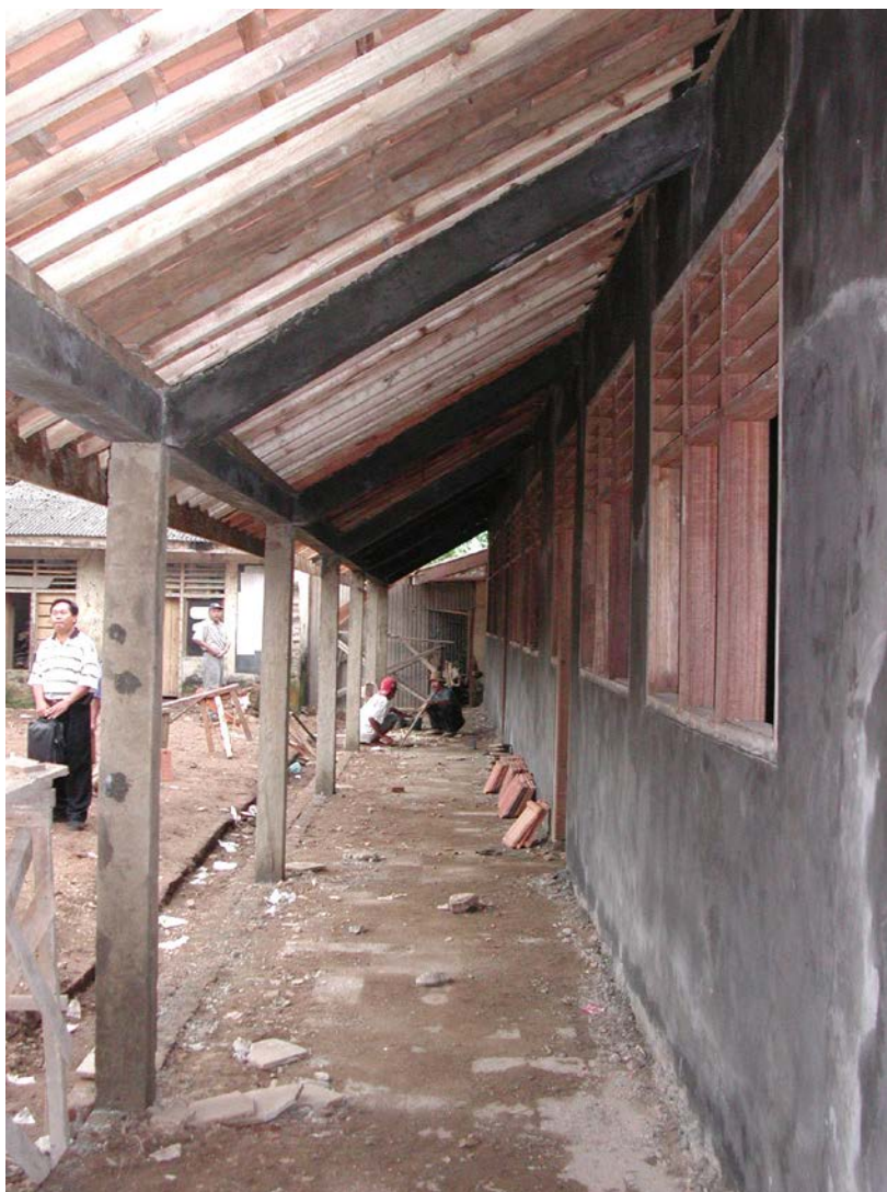
Plate 5: SDN Pandaj 1 showing veranda beams sitting over windows
