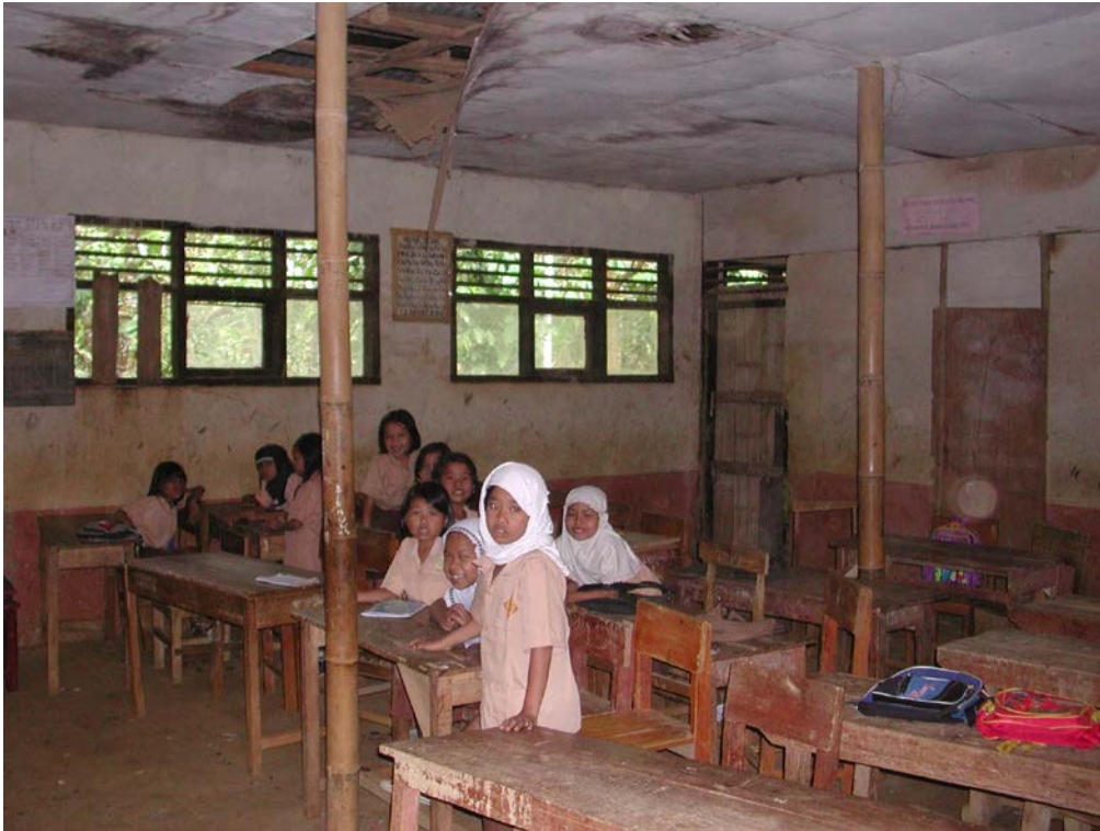
Plate 6: SDN Suka Raja showing interior of un-renovated building
