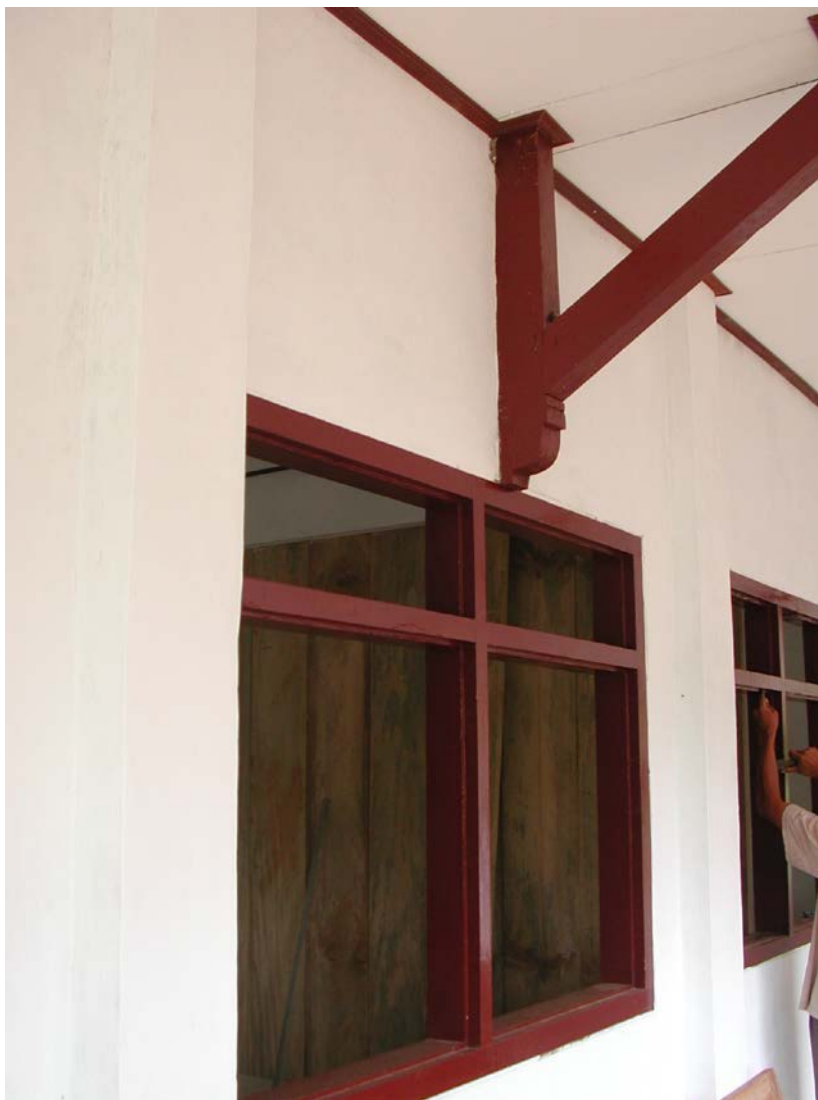
Plate 9: MTs Al-Fatah showing new roof trusses over windows
