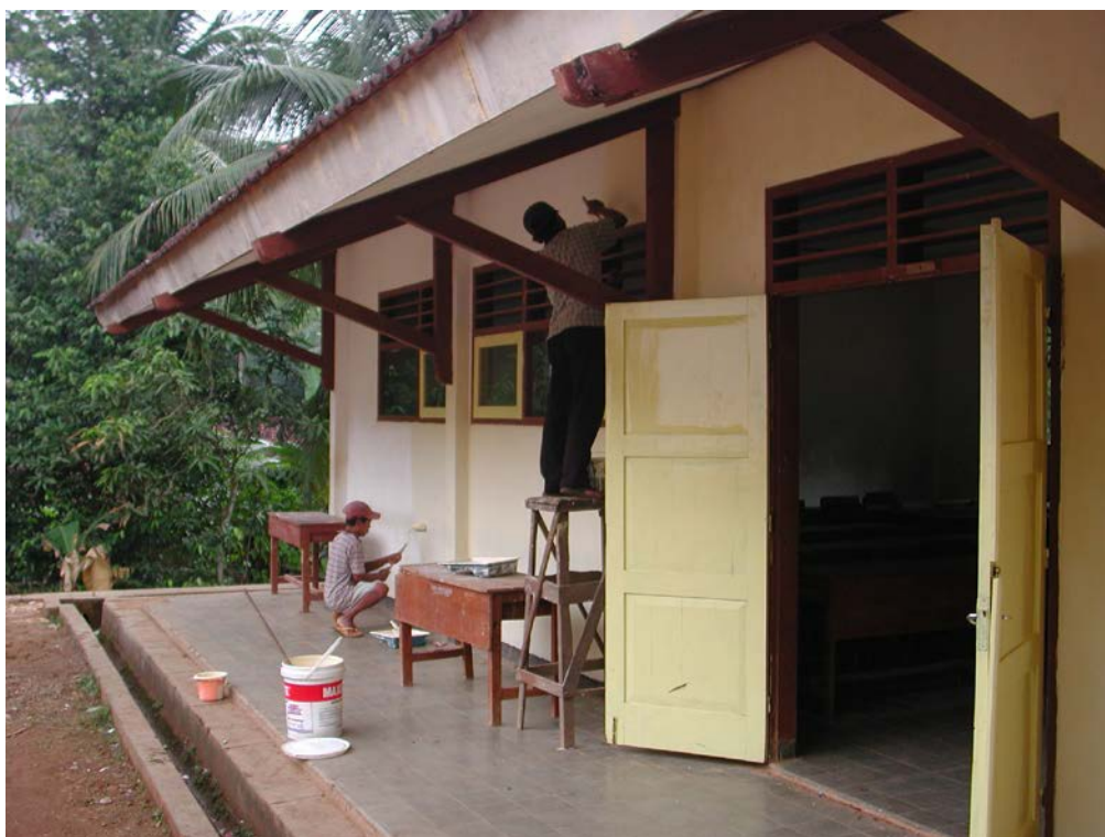
Plate 6: SLTPN Tegalombo showing renovations in progress
