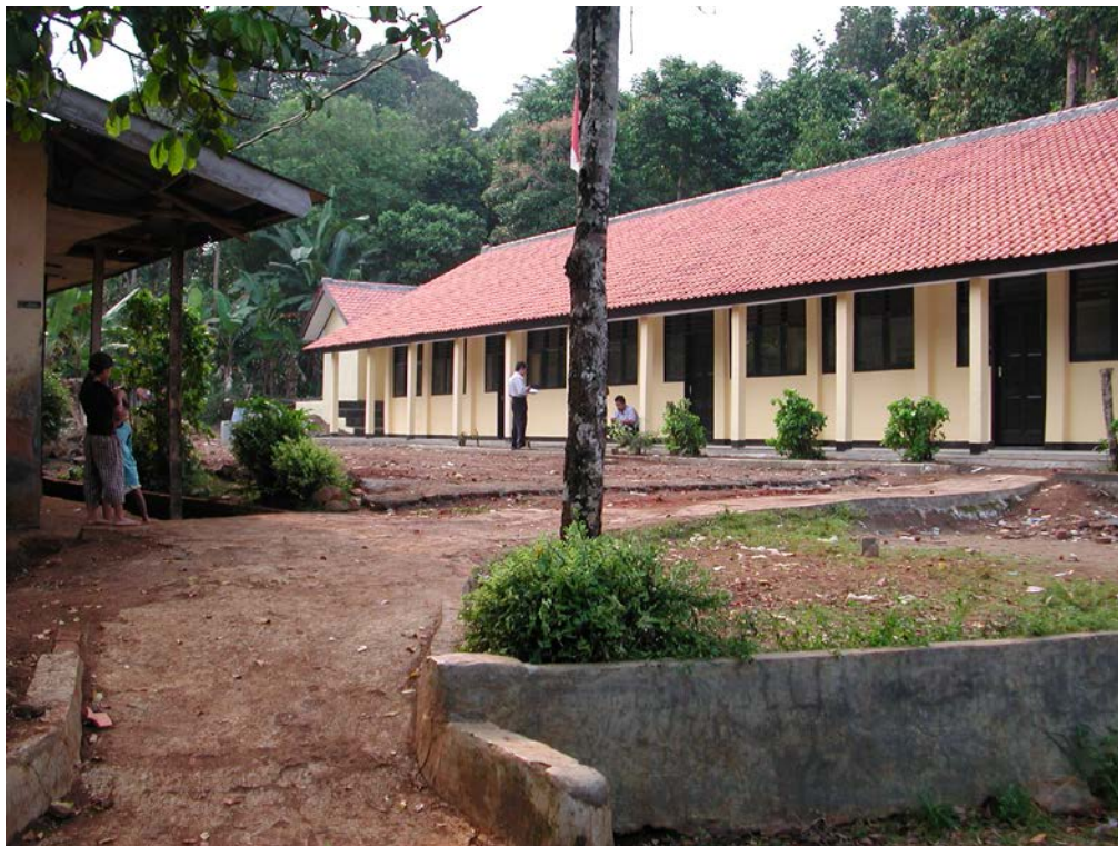
Plate 1: SDN Kadumerak showing new building with toilets at far end
