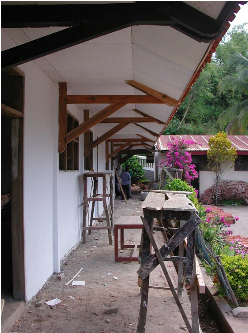
Plate 10: SDN Ploso 2 showing new building
