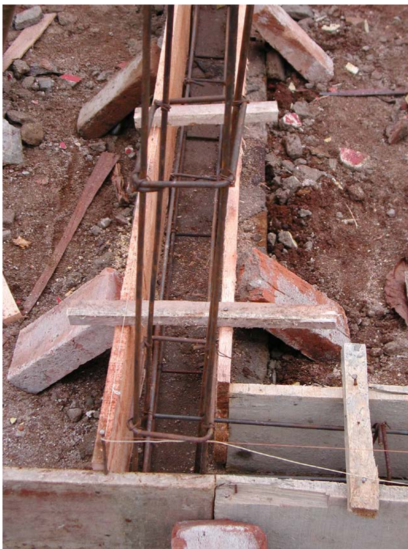
Plate 7: SDN Kerangi 1 showing 6mm reinforcement to office building
