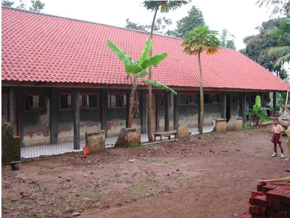
Plate 6: SDN Suka Raja showing renovated building
