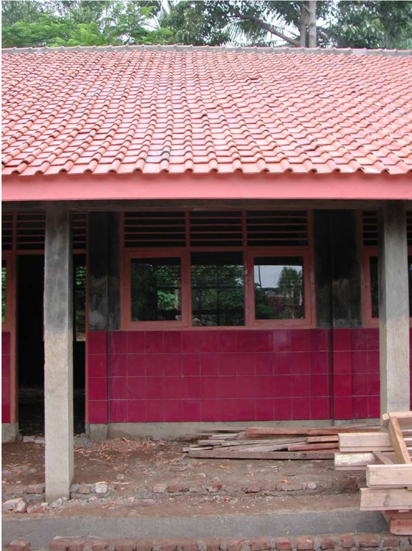
Plate 6: SDN Kerangi 1 showing renovated classrooms
