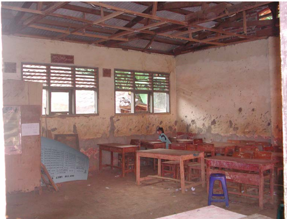
Plate 2: SDN Kadumerak showing inside of un-renovated building
