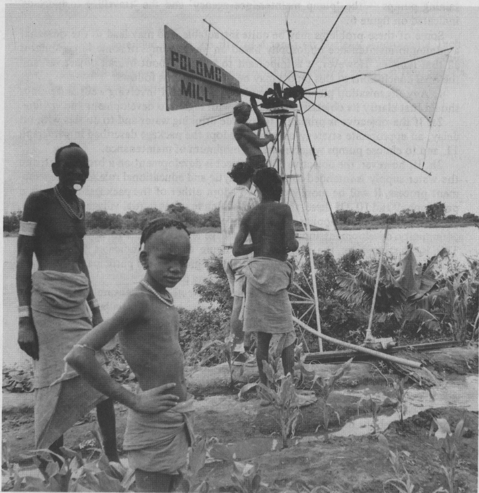
A typical "Polomo" Cretan-type windmill delivering water to a Geleb plot – the owner is on the left. Only four sails are deployed in this picture.
