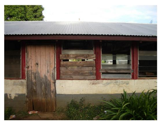
Plate 10: Classroom Building 4 showing generally poor condition and inadequate fixing of timber framing to walls.
