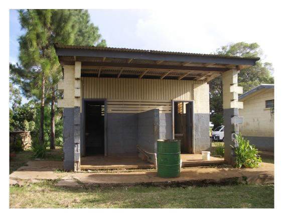
Plate 4: Toilet Building; note low pitched and poorly constructed roof
