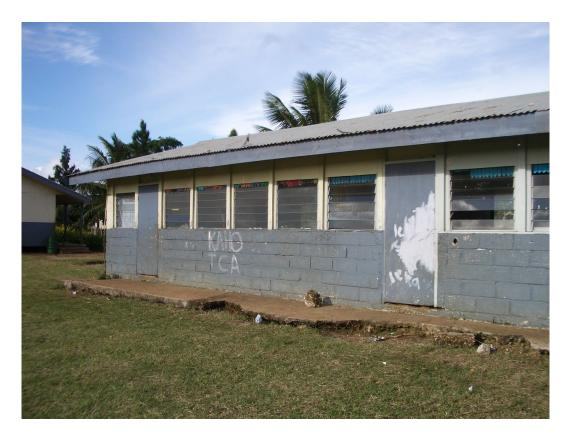
Plate 8: Classroom Building 4 showing poor condition and inadequate fixings to timber framing to walls
