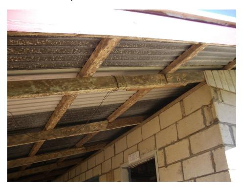
Plate 16: Inadequate roof structure and fixings to Classroom Building 2
