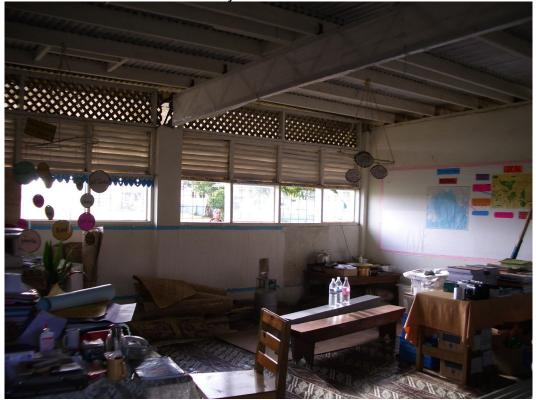
Plate 6: Classroom in Classroom Building 2 being used as an office; note wide spacing of purlins
