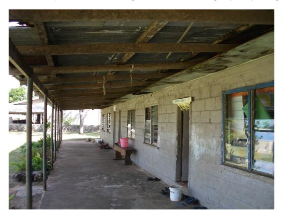
Plate 18: Rotting roof structure to veranda of Classroom Building 2
