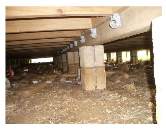
Plate 7: Foundation columns to Classroom Building 3 showing lack of bracing
