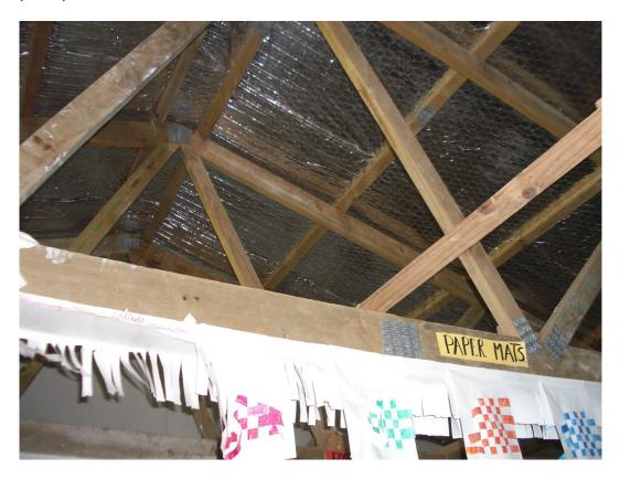
Plate 20: Inadequate fixings to roof timbers and wide spacing of purlins to Classroom Building 1
