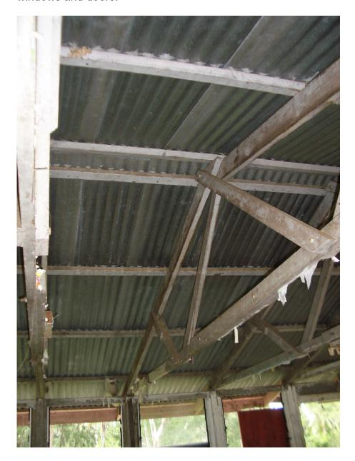
Plate 12: Inadequate bracing, purlin spacing and connections to roof timbers to Classroom Building 1
