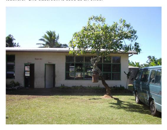
Plate 17: Classroom Building 1 showing large window area and lack of bracing in walls
