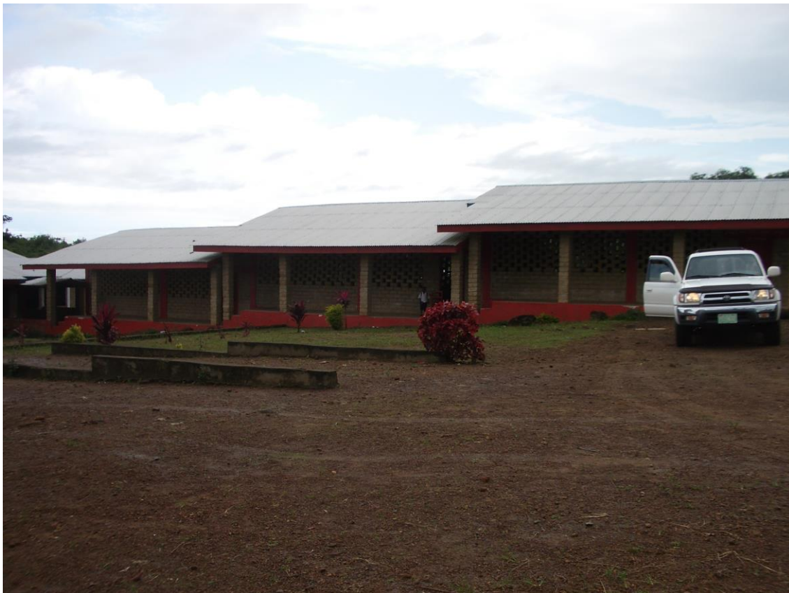
Plate 3: Kings Farm Public School showing one building stepping down the hillside and incurring extra foundation and roof costs
