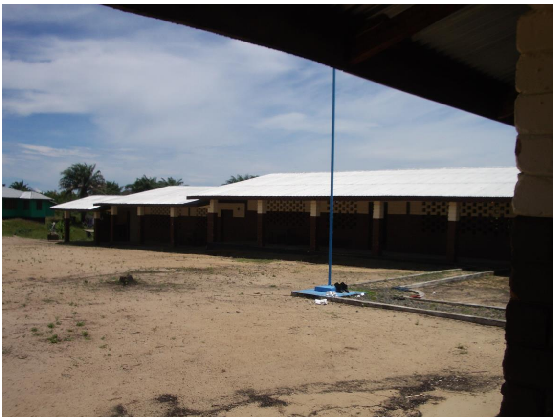
Plate 8: Duazon Blind Centre showing classrooms stepping down slope
