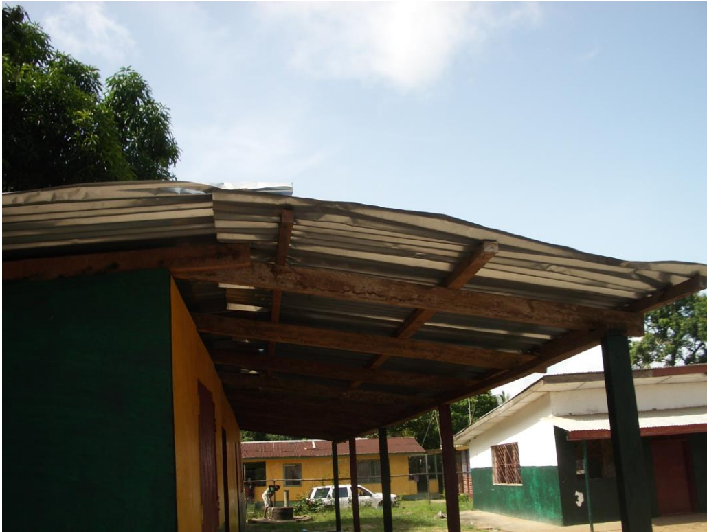
Plate 3: CAP Centre: close up of roof construction
