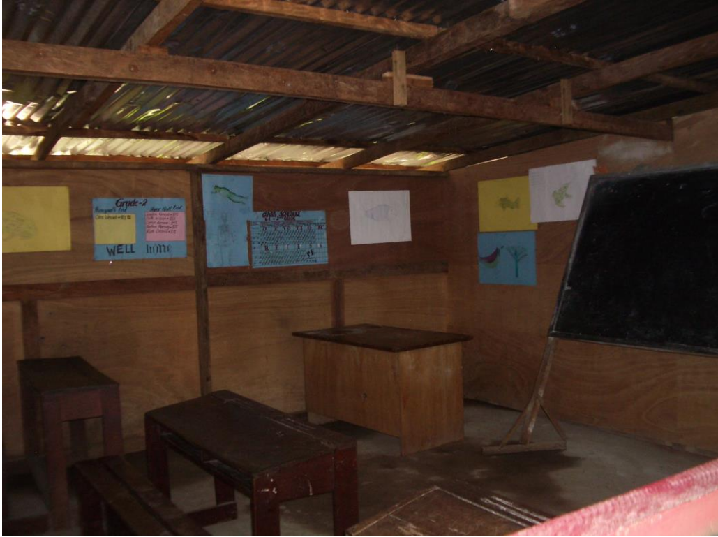
Plate 2: CAP Centre; internal view of activity room
