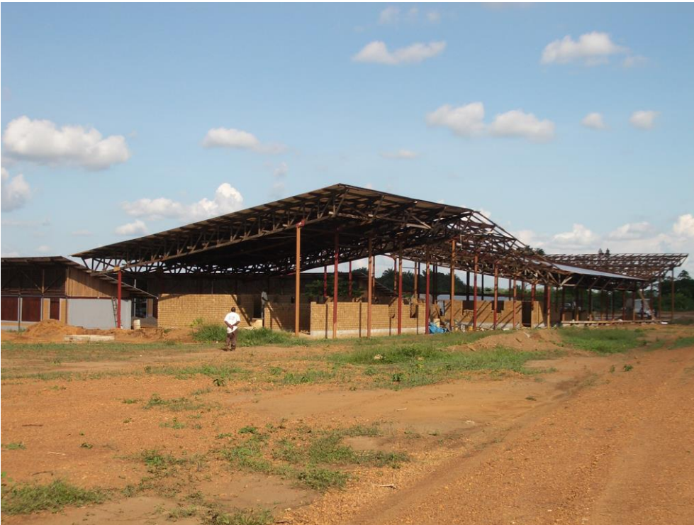
Plate 5: Ganta school showing steel framing and complex roof to community building
