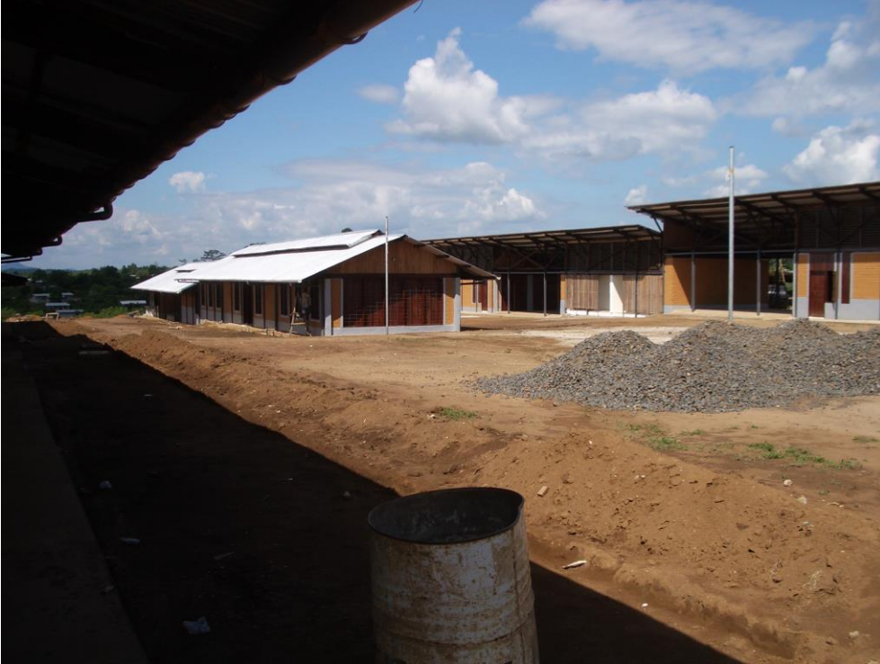
Plate 4: Ganta school showing the two types of classroom building. Note sun on walls and windows of building with mono-pitch roof.
