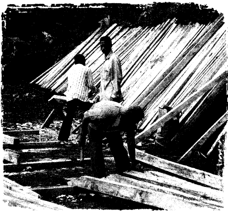
Key to success: identifying an experienced, knowledgeable and trustworthy coordinator or Kepala Pelaksana, like the one shown here at SDN Cijoho III in Kuningan, to manage construction and renovation work.
