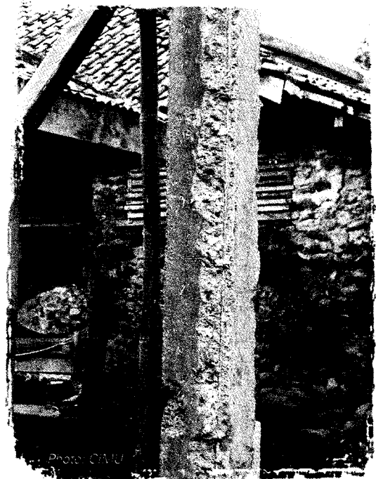
Poor quality concrete is easily identified. Advisors should be able to point it out and correct it during construction.
