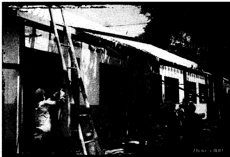
Local craftsmen replace the roof and veranda at SD Ketanggan 1 in Batang District, Central Java. These repairs were funded by the School Improvement Grants Program.
