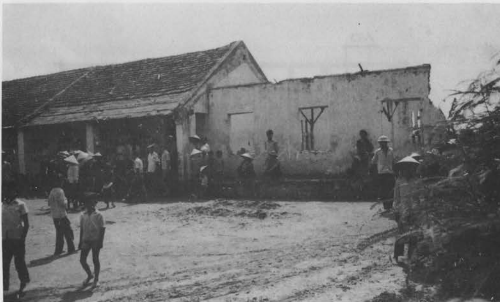
Fig. III.10 Rafters just placed on walls. Inverted trusses visible through windows.
