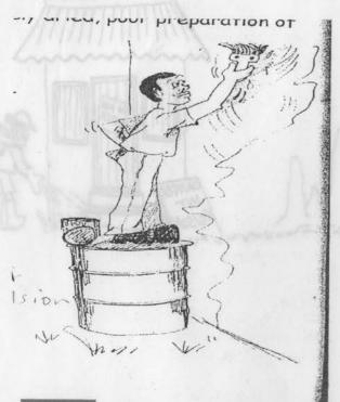
Solution for moisture in the wall, first you must remedy the cause. Refer to the section on damp proof course (see page 20). Strip the paint completely back to the plaster, ensure that the area is completely dried out, and repaint as follows. First apply one coat of good quality undercoat, followed by a minimum of two coats of good quality gloss or emulsion paint as required.
