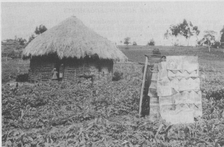
Plate 2. A simple pit latrine in rural Kenya. A latrine of this sort may be quite acceptable for many years but tends to become smelly and to attract flies. It may be improved by adding ventilation as shown in Plate 1. (Photo: R. G. Feachem).
