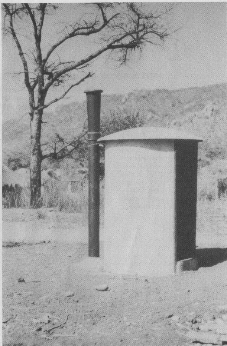
Plate 1. A ventilated pit latrine in rural Zimbabwe. Improved pit latrines of this type provide a low-cost, hygienic, odour free and acceptable excreta disposal system which is appropriate in many rural settings. (Photo: V. de V. Clarke).
