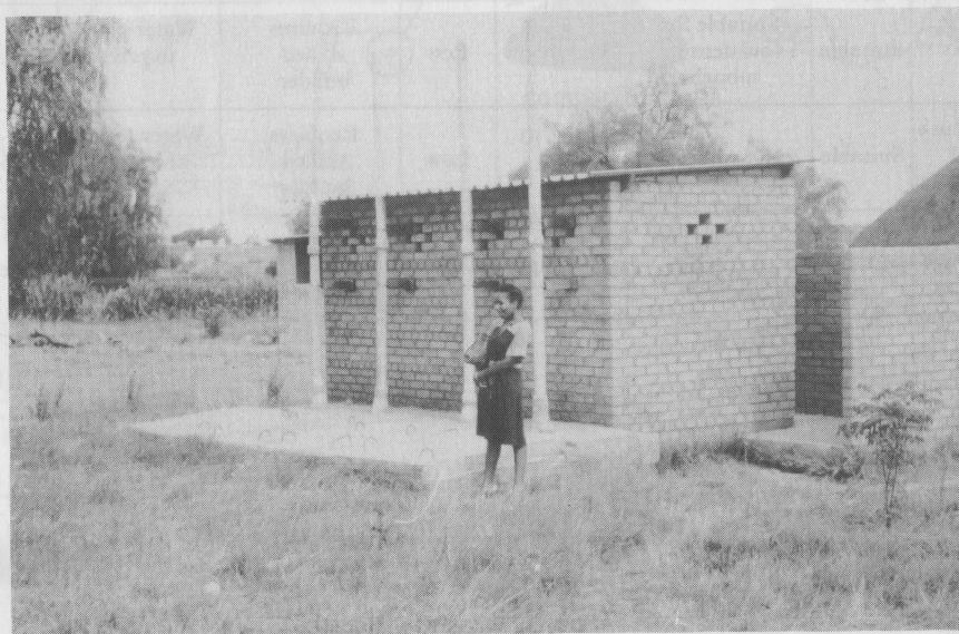
Plate 7. The back of four ROEC offset pit latrines in Botswana. The large ventilated pits are under the concrete slabs. The vent pipes should be black. (Photo: R. G. Feachem).
