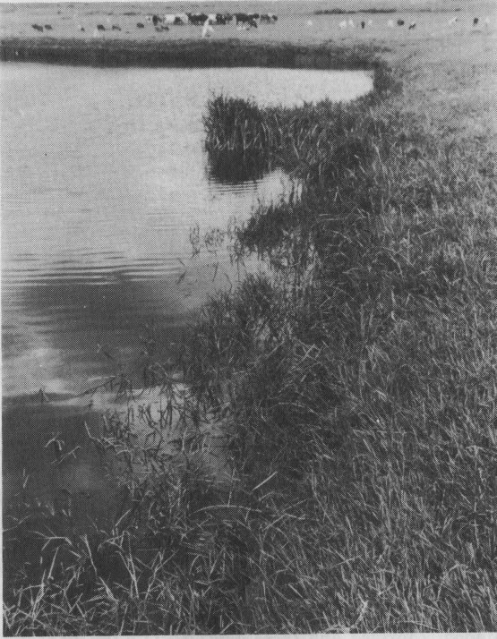
Plate 10. Two waste stabilization ponds. The banks of pond 1 are not properly constructed and extensive colonization of the pond by vegetation is taking place. This will reduce the pond volume and allow snail and mosquito breeding near the shore. The pond is unfenced and there is nothing to prevent the cattle from drinking from, or wading in, the pond. Pond 2 is well constructed and the banks are clearly being kept clean. A simple inlet arrangement is also shown. (Photos: D. D. Mara).
