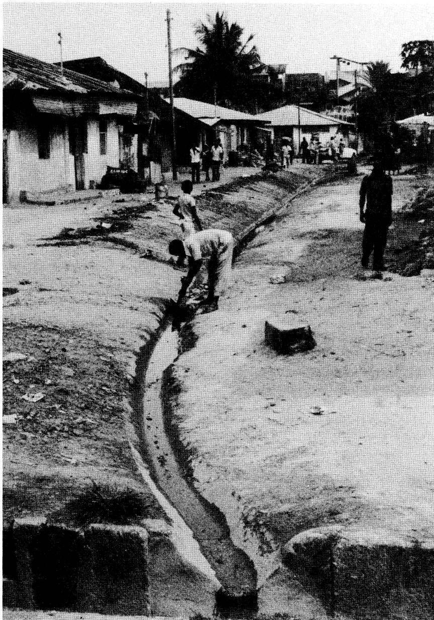
Open drains provide places for insect breeding as well as allowing access to polluted waste water for children and animals
