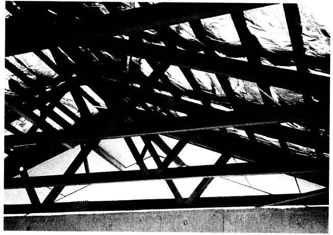
Figure 5 Use of nail plates in roof construction
