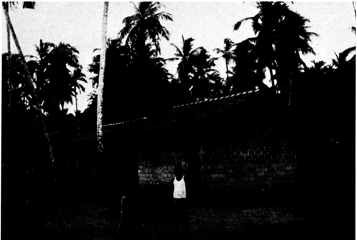
Sri Lankan village houses, built from blocks of cement-stabilised soil
