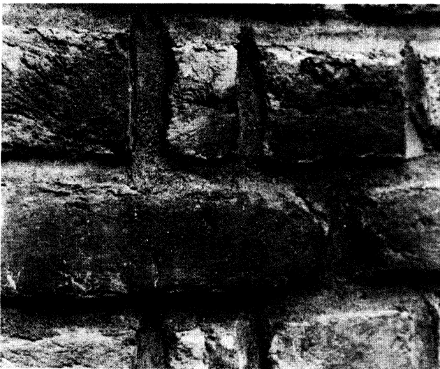
Figure 16 Rice husk ash cement used in mortar in India
