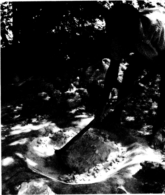
Figure 17 Gypsum plaster and aggregate being mixed in Cape Verde
