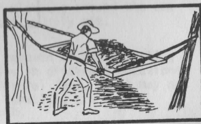
Fig. 5 - Screening the Soil.
