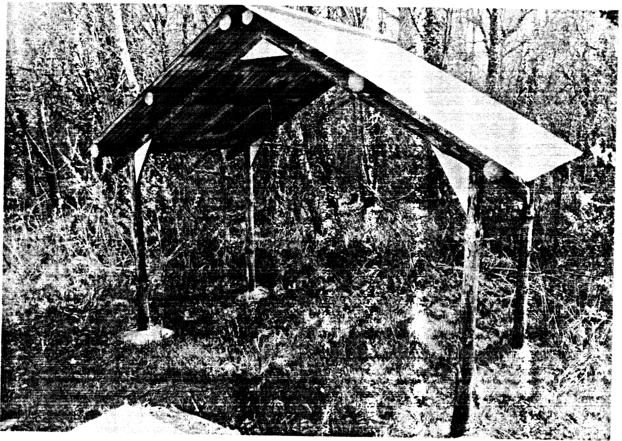
Plate 7 Portal frame structure at BRE.
