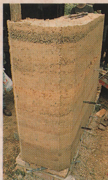
Above: rammed-earth wall detail
