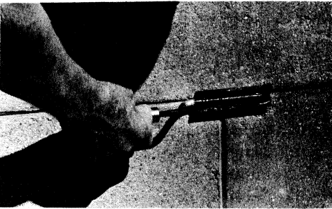
V joint being formed with special V tool.
