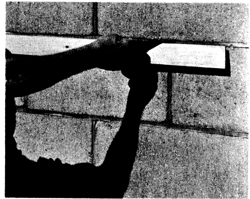
Weatherstruck joint being formed with a straightedge and frenchman.
