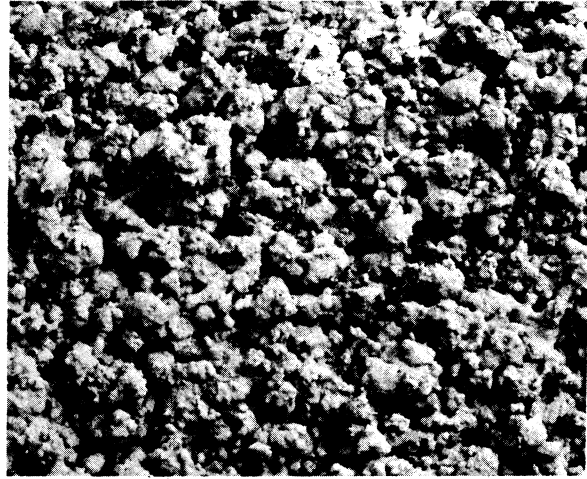
Fig. 24. Machine-thrown finish: coarse texture (approx. full size).
