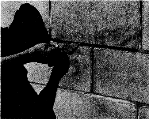
Struck joint, mortar compacted with trowel stroke.
