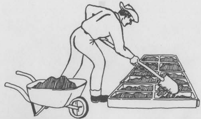
Figure 39. Charging the forms.
