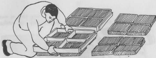
Figure 41. Lifting the forms from freshly made blocks.
