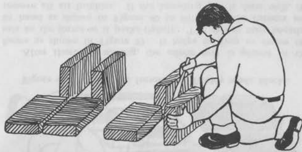
Figure 45. Unstabilized block is turned on edge to dry after two to four days.
