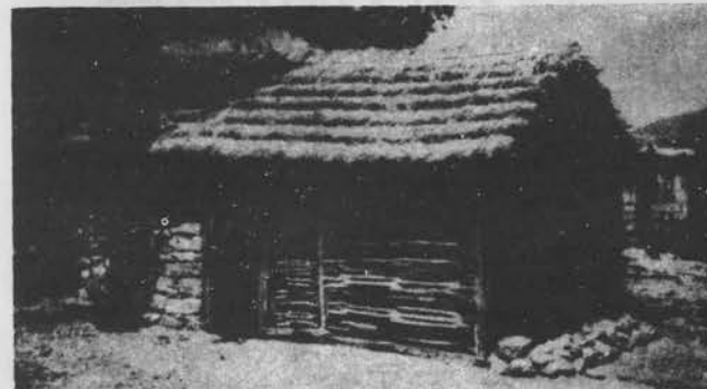
Figure 4. The right half of this residence in Greece shows the wattle in place. Daub will follow.
