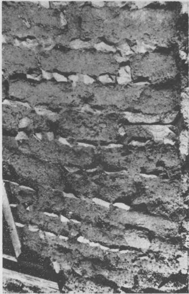
Figure 63. The mechanical bond of plaster to the adobe wall was enhanced by the early builders of Ft. Davis, Texas, by inserting rock chips in the fresh mortar.
